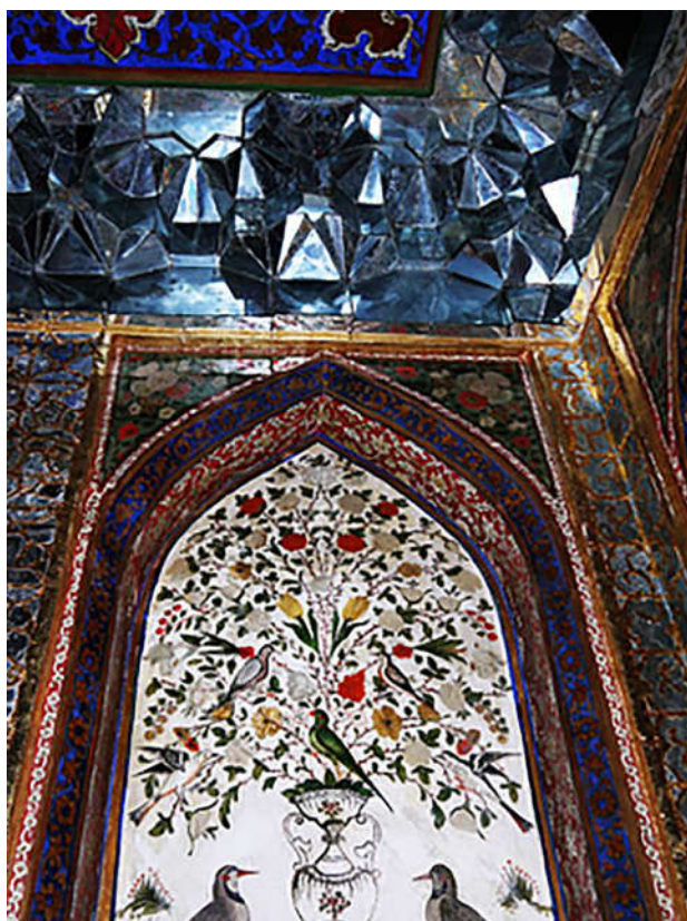
Fig. 7. Mirrored ceilings, shebeke, paintings and a ventilation fireplace in the interior of the Sheki Khan's Palace (protected by UNESCO) Photo of the site // https://myslo.ru/club/blog/gulbarij/PBa-pgmDHkCdFYc3VLNBlw .
