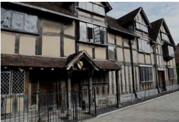
Figure 4. J. Shakespeare's town half-timbered house, Stratford. 16th century Source: (Brisco T.)
