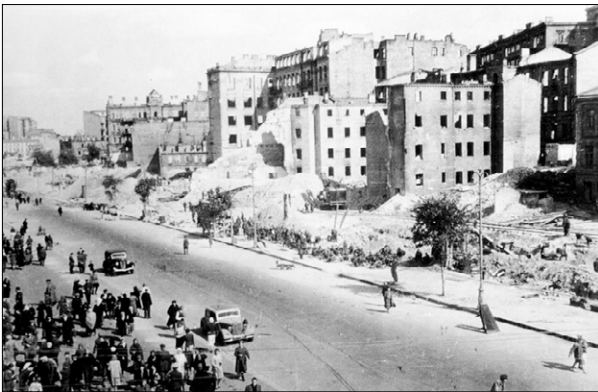
Fig. 7. Remains of the Ginzburg House, 1941; source: collection of the Malakov family
